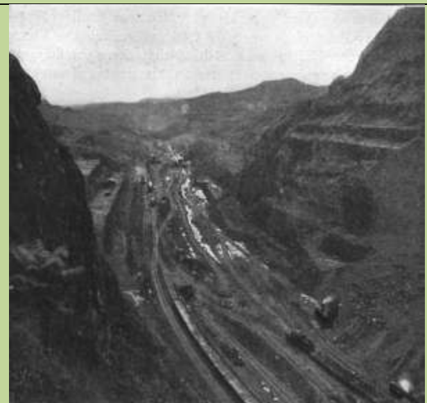
Deepest Excavated Portion of Panama Canal, Showing Gold Hill on Right and Contractor's Hill on Left. June, 1913
