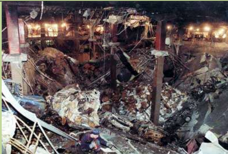
Damage from 1993 World Trade Center Attack
