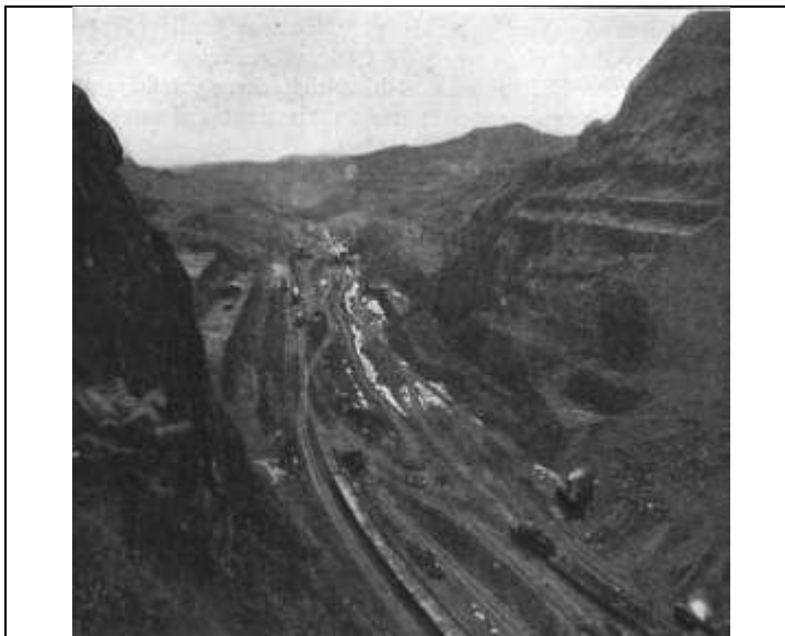
Deepest Excavated Portion of Panama Canal, Showing Gold Hill on Right and Contractor's Hill on Left. June, 1913
